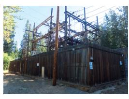
The Brockway substation is about 50 years old and has reached the end of its useful life. Brockway experienced numerous problems during the winter storms earlier this year. Replacement and/or repair of existing parts are unfeasible and not cost effective.
